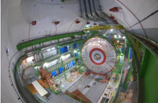
Installation of a 1270-ton component of the CMS detector for the Large Hadron Collider, which physicists hope will detect the Higgs boson of the Standard Model.
